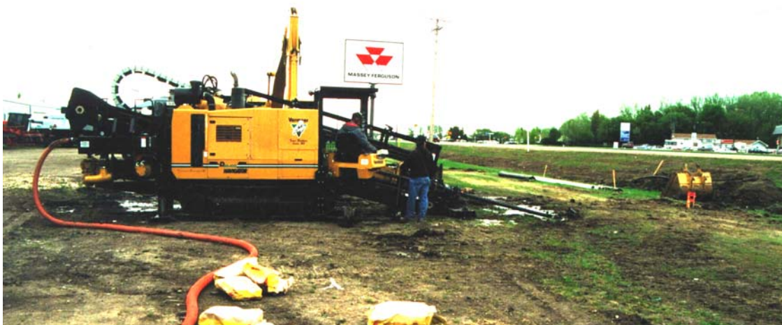
Pipeline is tunnelled under highway.
