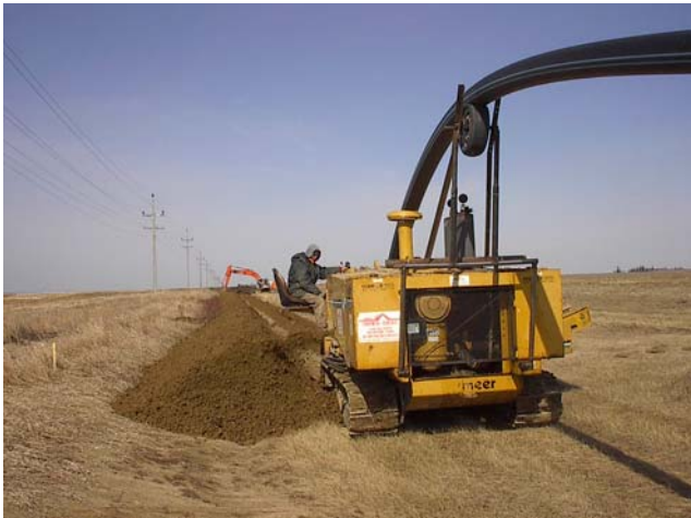
Trencher installs pipeline.
