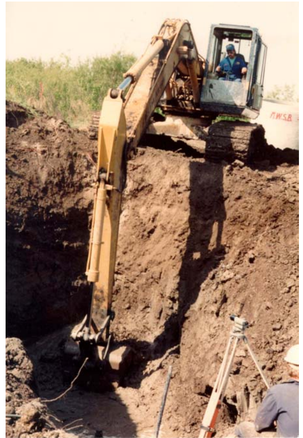
Backhoe installs wet well
